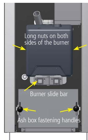
Burner cleaning is started by unfastening the long nuts on both sides of the burner and by pulling the burner out of the boiler. Make sure that the burner wires do not get damaged.
