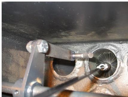
5. Sweep the convection tube surfaces with a round brush and remove fly ash. Insert the brush all the way down and lift back up.
