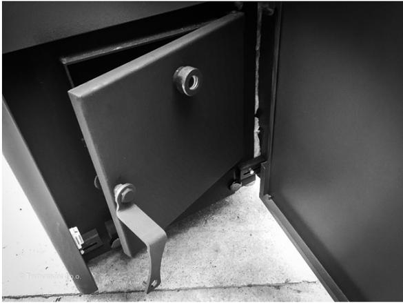
Open the lower, chamber door with the boiler KEY.
