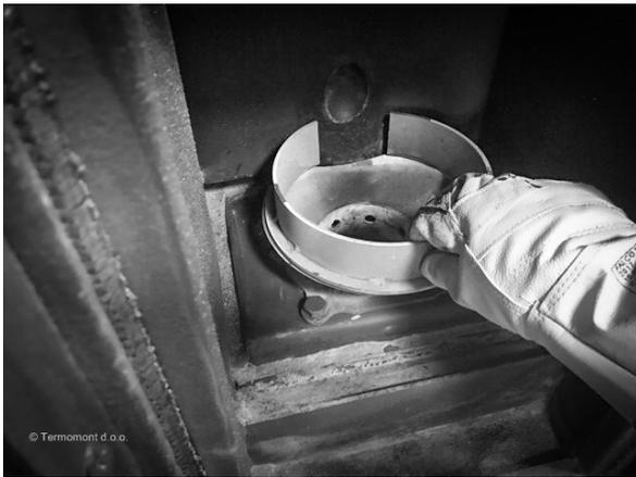
Put the upper burner part back in place.
