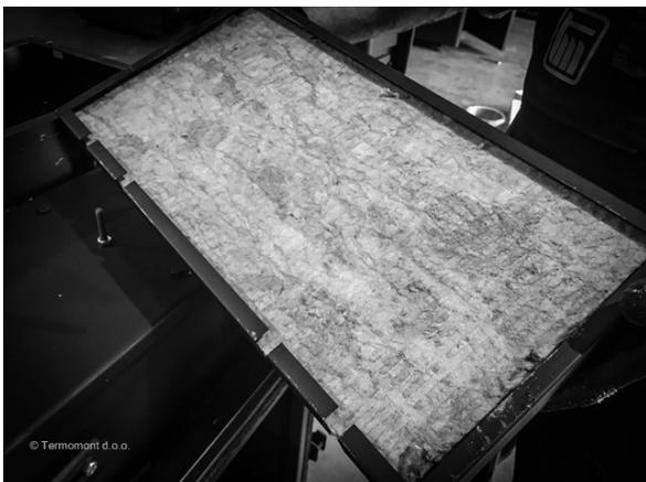
make sure you make no damage to the stone-wall insulation below.
