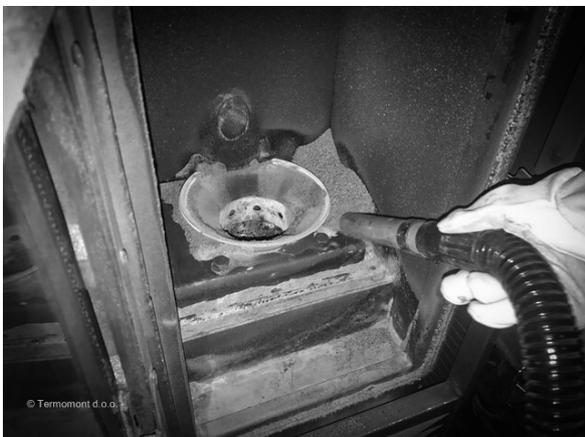
Clean the area around the burner. If you don't have an ash vacuum cleaner, use the manual tools that are delivered with the boiler.
