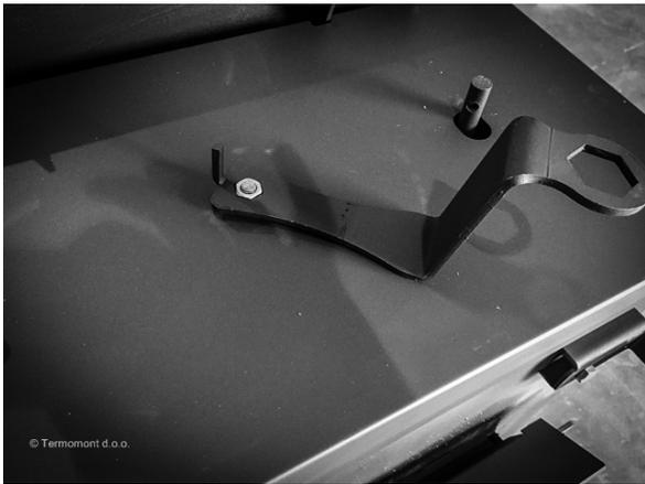
The insulation coat is attached below this metal cap. To unscrew the cap use boiler KEY.
