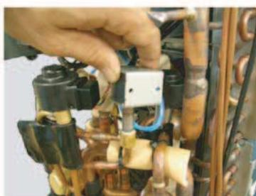
Remove the SOLENOID COIL.
