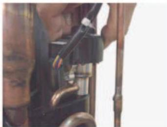
Remove the EEV coil by hand.
