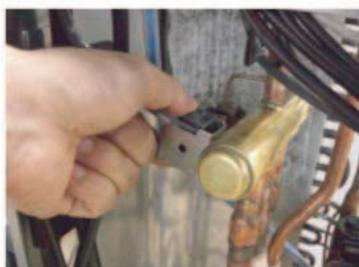
Remove the SOLENOID COIL.
