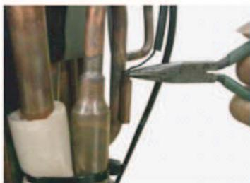
Remove the THERMISTOR SPRING.
