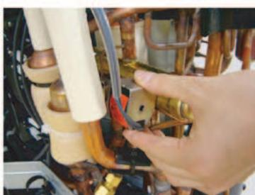
Remove the SOLENOID COIL.
