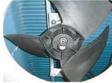
Remove the Hex Socket Screw and remove the PROPELLER FAN.
