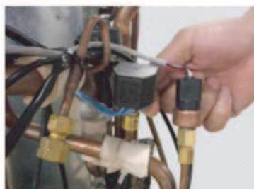
Remove the SOLENOID COIL.
