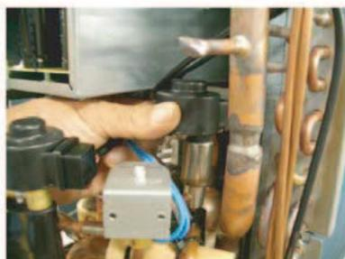
Remove the EEV coil by hand.
