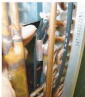
Remove the THERMISTOR SPRING.
