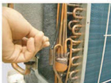
Remove the THERMISTOR SPRING.
