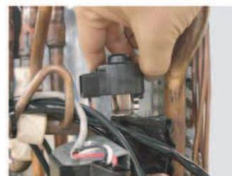
Remove the EEV coil by hand.
